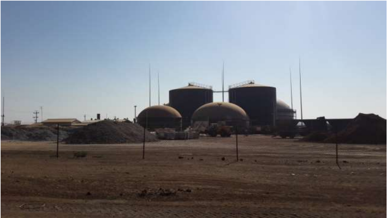
Figure 18: Bio2watt plant near Bronkhorstpruit, South Africa
